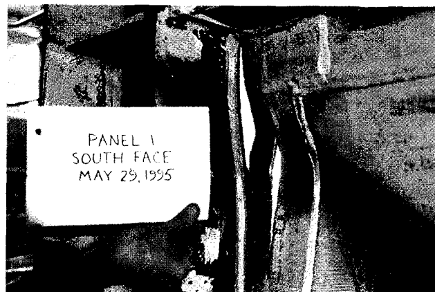
FIG. 3. Tears at Top West Corner of Panel 1
